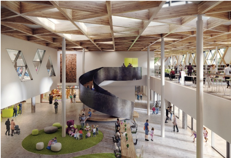
Beneath the canopy is an inside space that strives to be responsive and evolving, both physically and with its activities. (Image: HCMA Architecture + Design)
