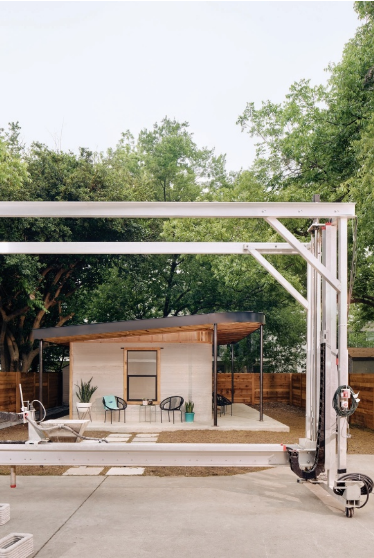
A 3D-printed home in Texas, created with ICON's Vulcan printer, may be a precursor to solving housing shortages throughout the globe. (Image: ICON)
